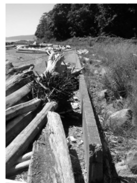
Ala Spit Seawall
